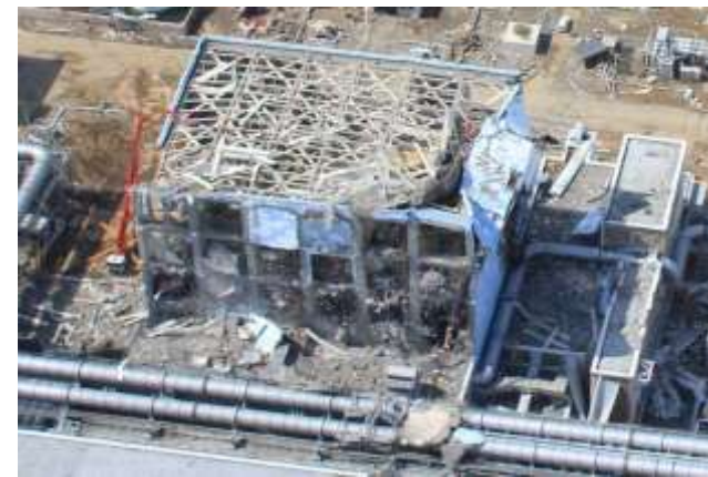
Reactor No. 4 (East side) Hydrogen built up in the 5 th & partially in the 4 th , floor (east west)
