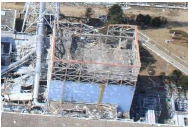
Reactor No.1 (East side) Hydrogen built up in the 5 th floor
